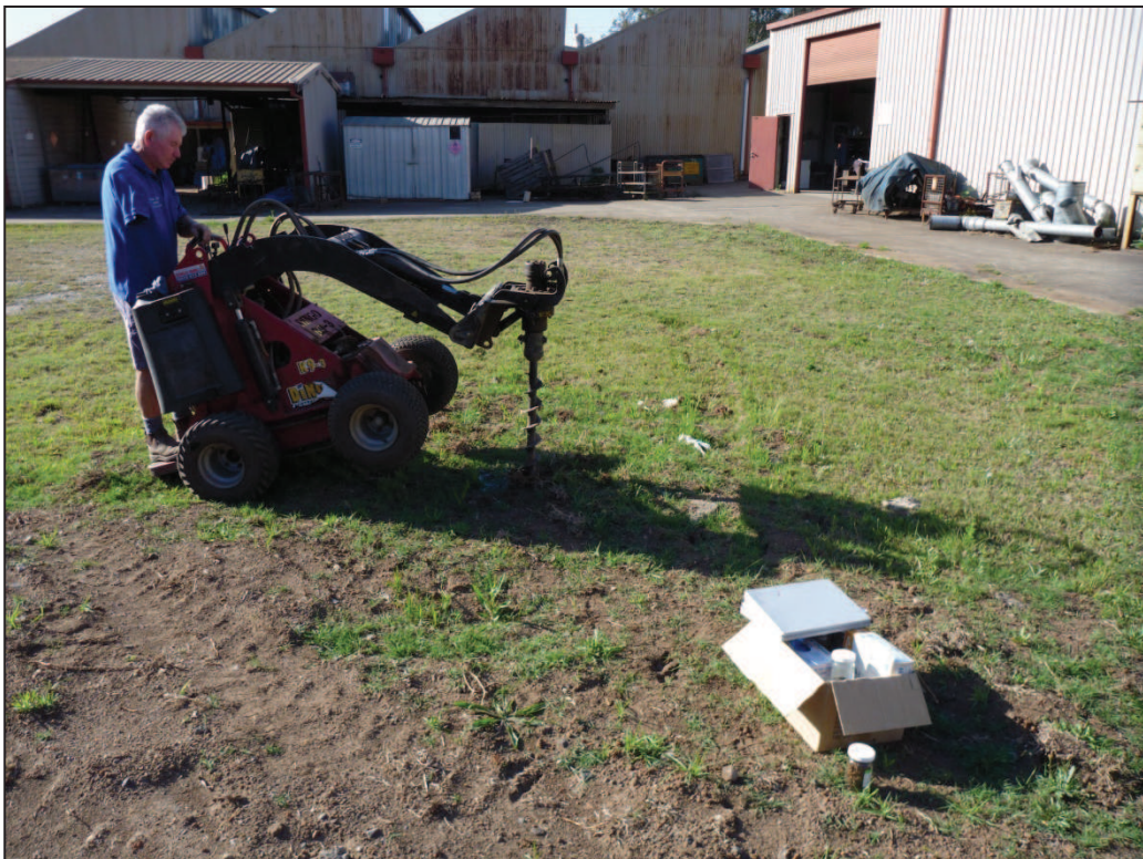
Plate 32 – Boring location B5.
