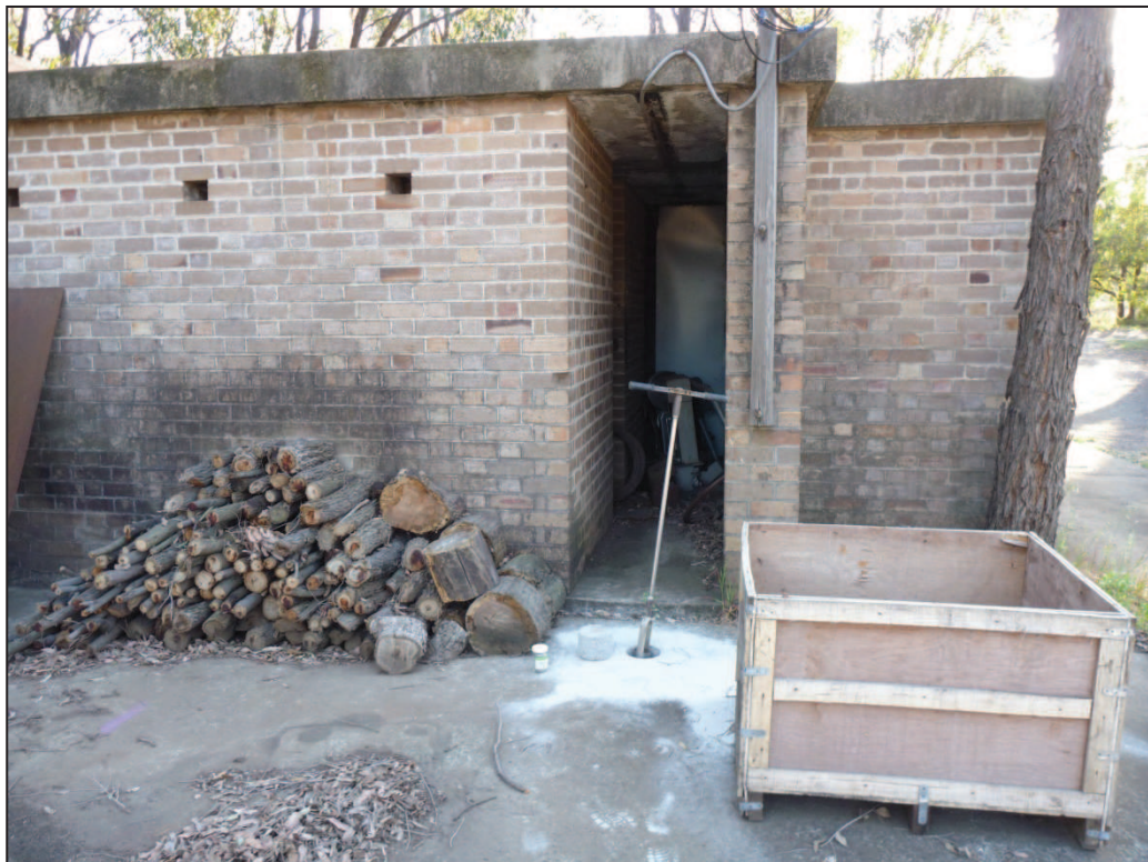
Plate 40 – Boring location B15.
