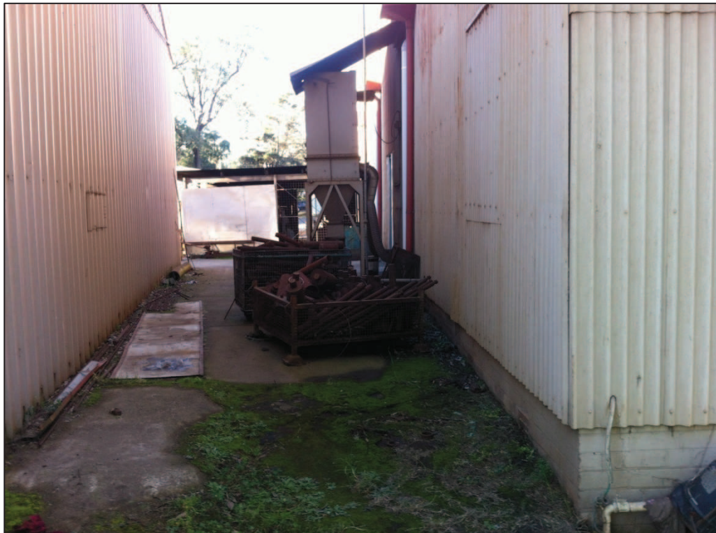
Plate 13 – Locations 16 and 17, scrap metal and a hopper (part of air extraction system for Coils Factory) between the Leaf Springs Shed and Coils Factory on the southern portion of the site.
