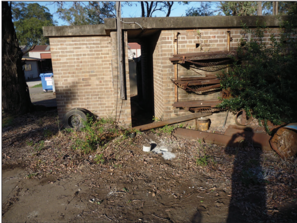
Plate 39 – Boring location B14.
