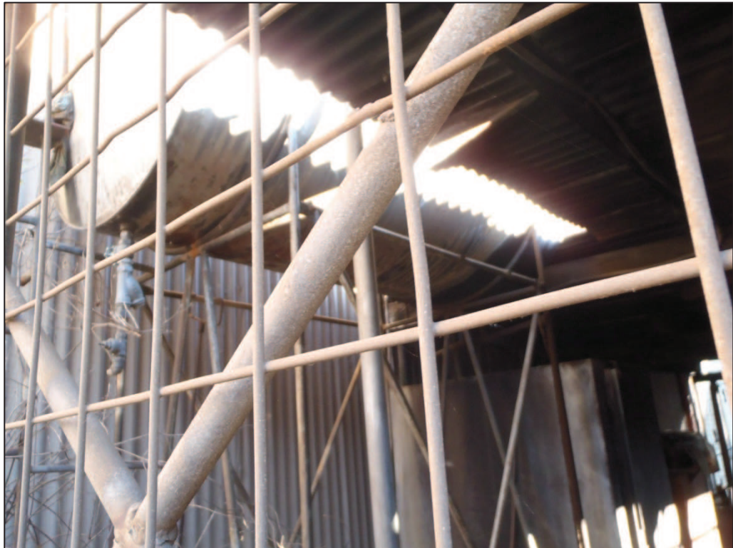
Plate 22 – 2,500L diesel AST (AST 3) adjacent north of the eastern portion of the Coils Factory (Location 27).
