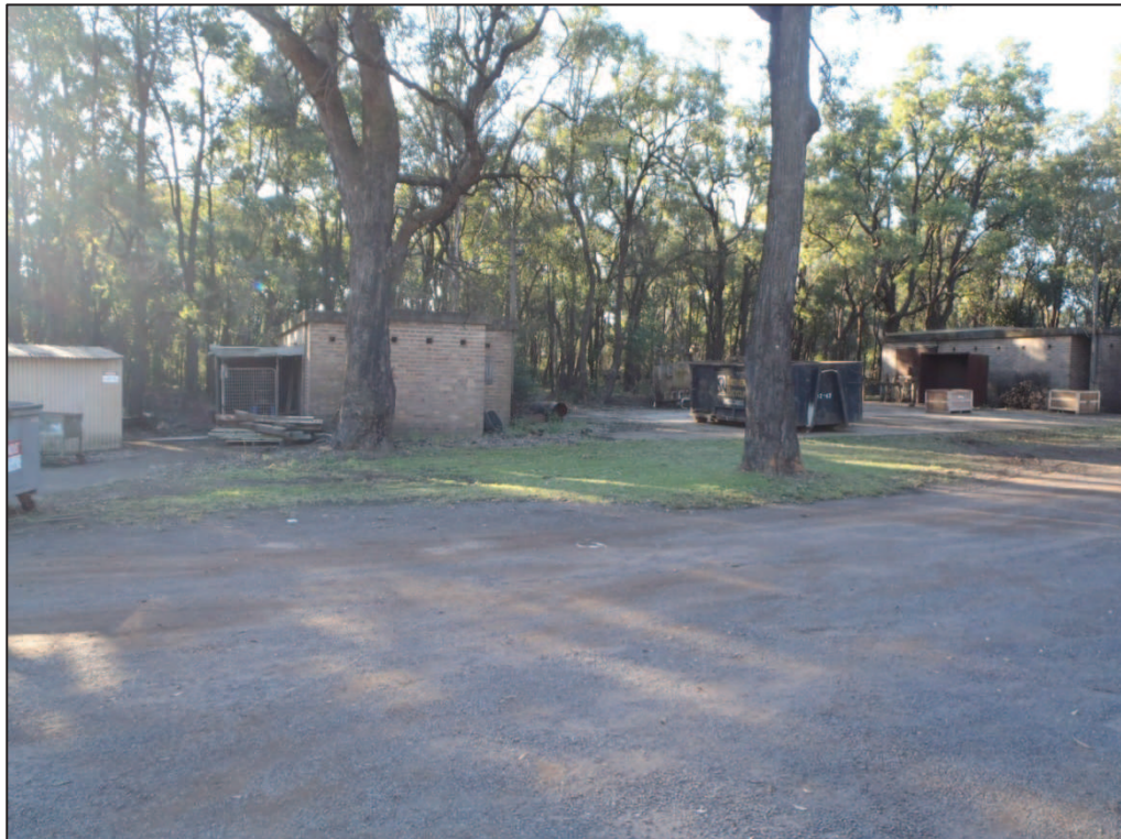
Plate 15 – The old ammunition bunkers on the eastern portion of the site.
