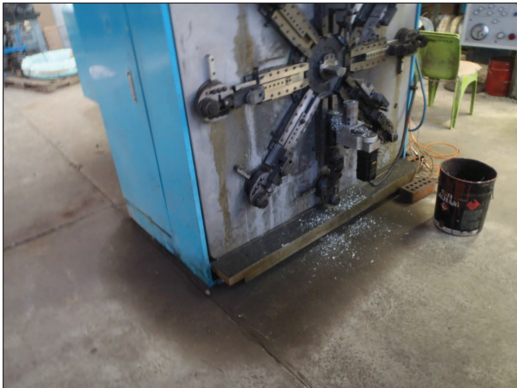
Plate 30 – Dark staining around machinery in the eastern half of the Coils Factory.
