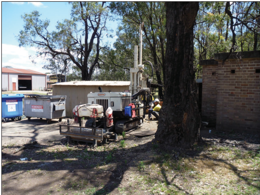
Plate 42 – Boring location B17.
