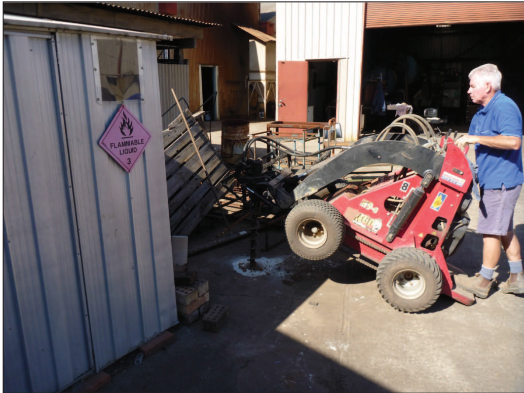
Plate 35 – Boring location B8.
