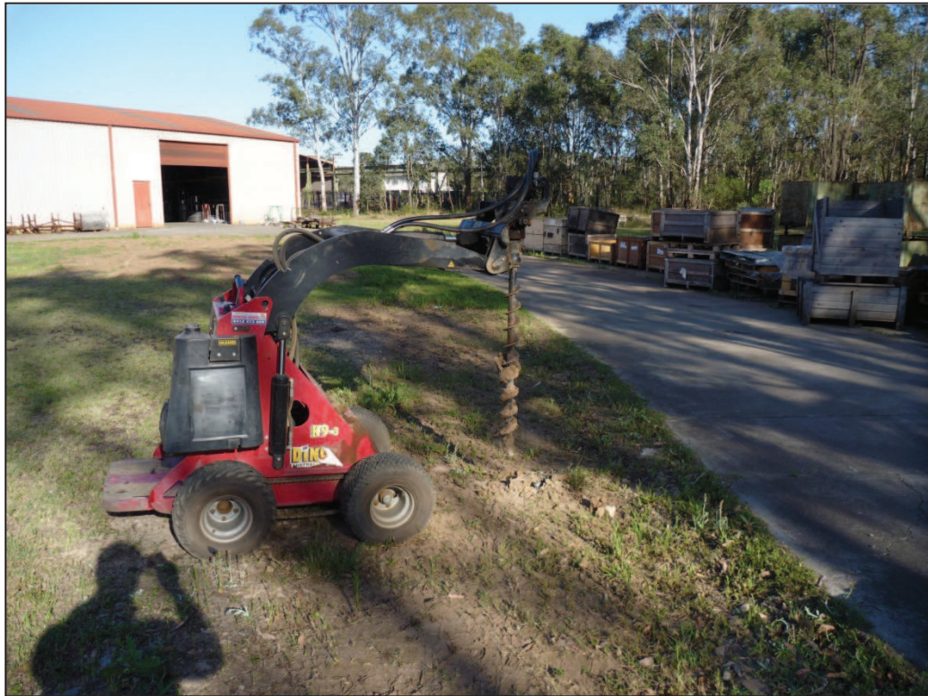
Plate 33 – Boring location B6.
