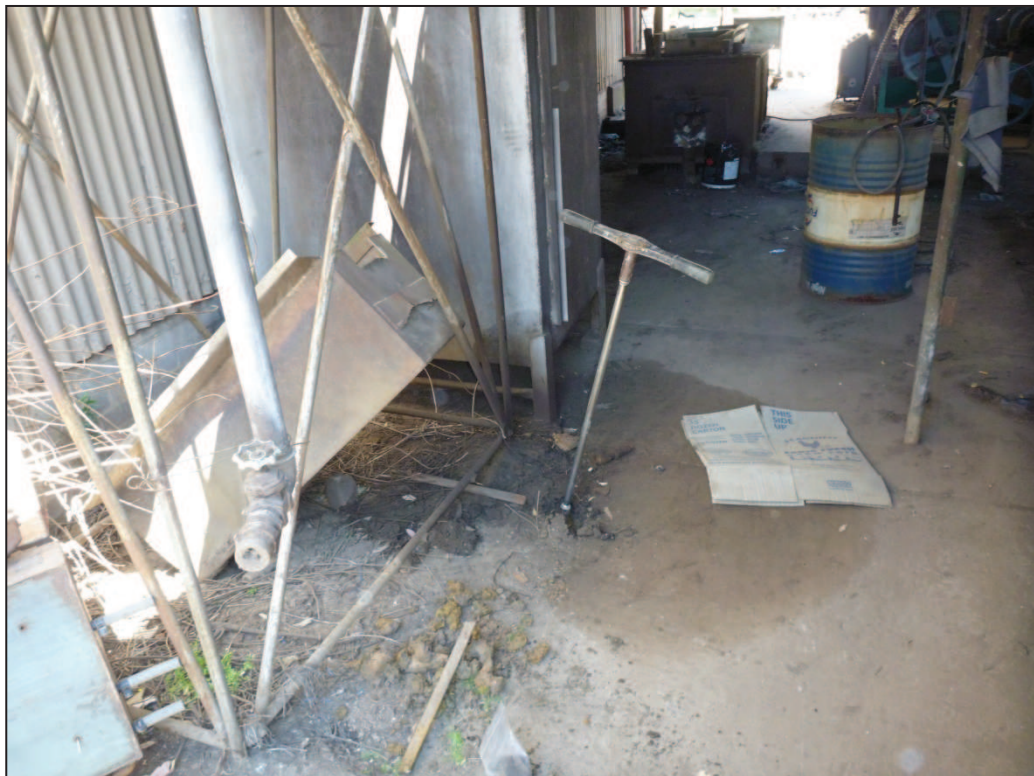
Plate 50 – Boring location B24.
